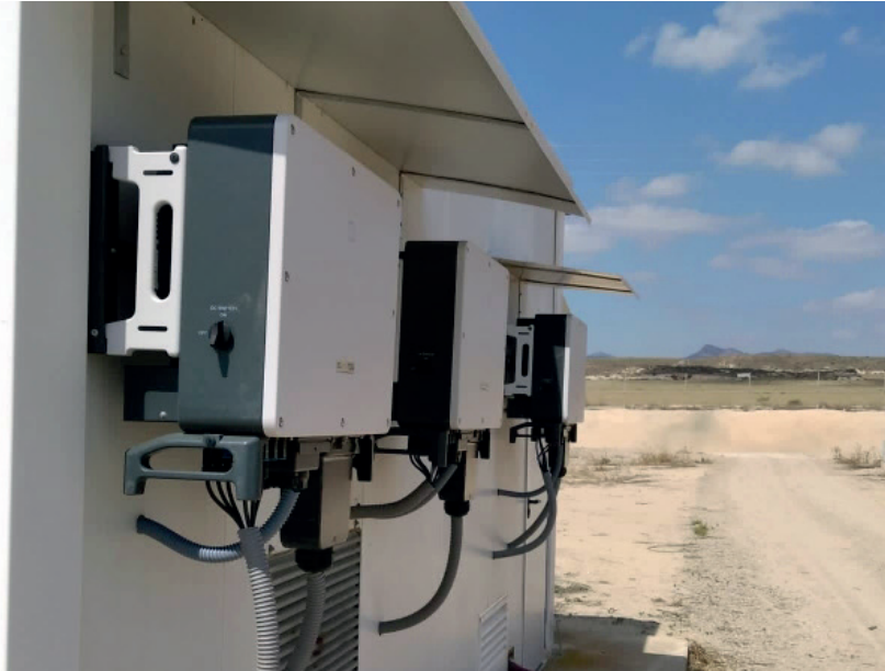
SG33CX are IP65 and can be placed outdoor.
